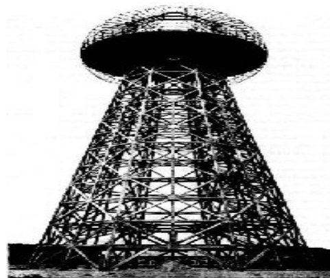
Fig.1. The 187-foot Wardencllyffe Tower (Tesla Tower) in 1903. This was to be the first broadcasting system in the world. Tesla wanted to transmit electricity from this Tower to the whole globe without wires using the Ionosphere. The source of the transmitted electricity was to be the Niagara Falls power plant[1].
